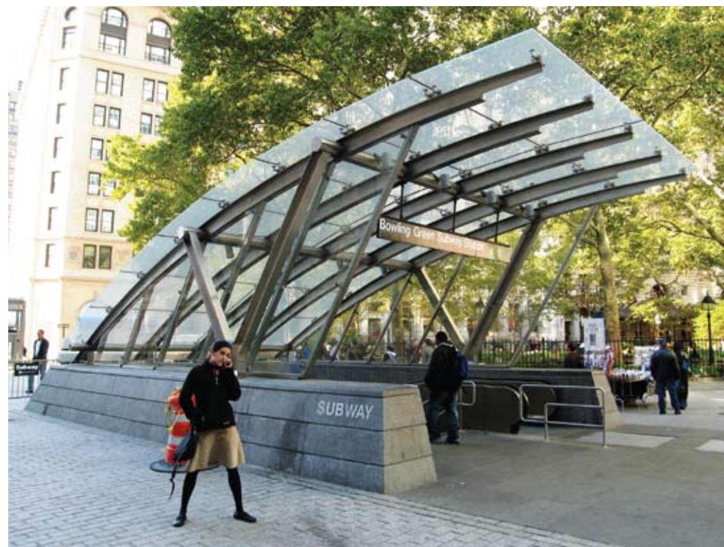
Bowling Green Station , New York, NY, Dattner Architects
