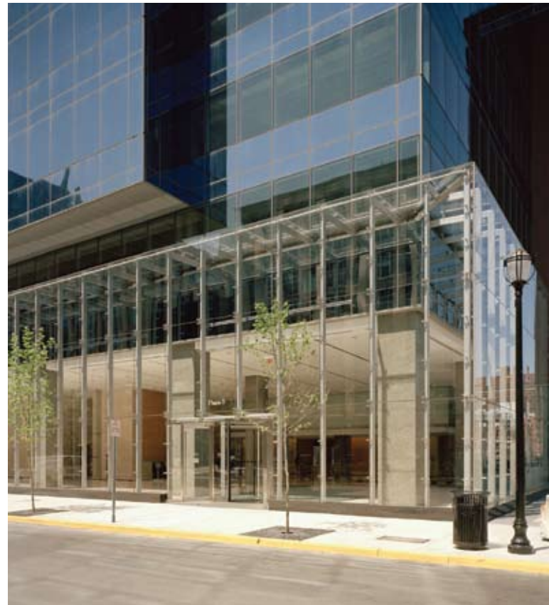
Harborside Financial Center , Plaza 5, Jersey City, NJ, Grad Associates
