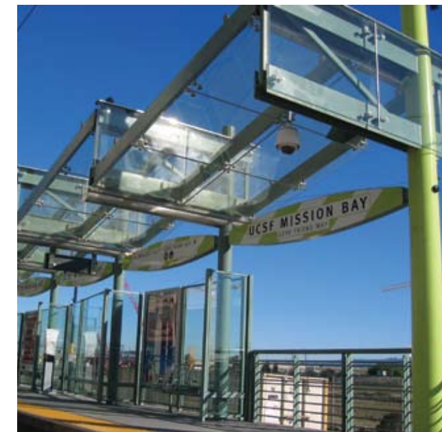
3rd Street Light Rail , San Francisco, CA City of San Francisco Bureau of Architects
