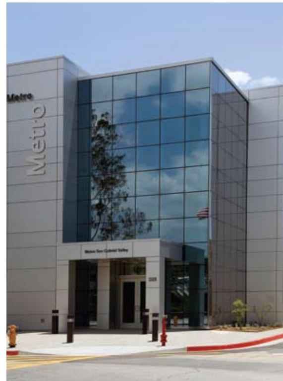
TOP: Las Vegas Motor Speedway , Las Vegas, NV, ai Design Group BOTTOM: Metropolitan Transit Authority , Division 9 Transportation Building, Los Angeles, CA, Designer: MTA
