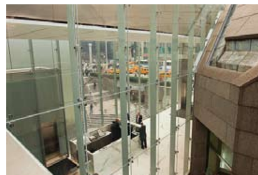
Side mounted spider stainless steel castings and Planar 902 countersunk fittings attach the laminated glass to the vertical plate beams.
