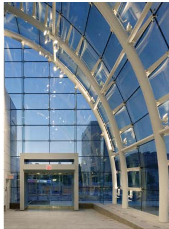
TOP: Park Tower Lobby, Costa Mesa, CA, Murphy Jahn Architects BOTTOM: Pier 79 West Midtown Ferry Terminal, New York, NY, William Nicholas Bodouva + Associates
