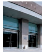
Page 23 Santa Ana Police Administration & Holding Facility Santa Ana, California Architect: Hellmuth, Obata & Kassabaum
