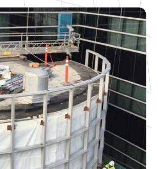
With installation training provided by EFCO, the glazier was able to assemble the new curtain wall in front of the existing brick facade. CASE STUD'
